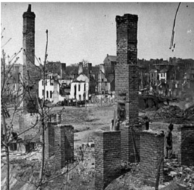
Chimneys standing amidst rubble
