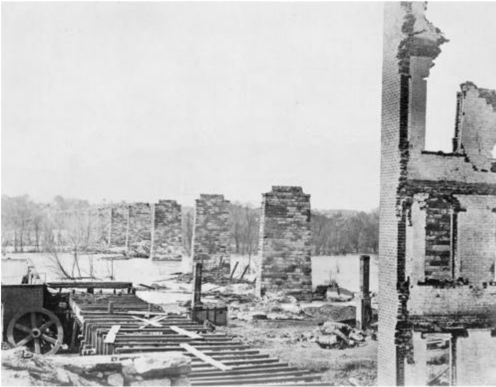
Richmond and Petersburg Railroad ruins of bridge
